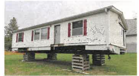
FGCI purchased a used double-wide manufactured home that will soon serve as an annex to the Camp of the Good Shepherd chapel, providing restrooms, a kitchenette and a meeting room.
