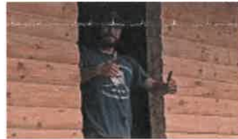
Collier in the opening for the new window.
